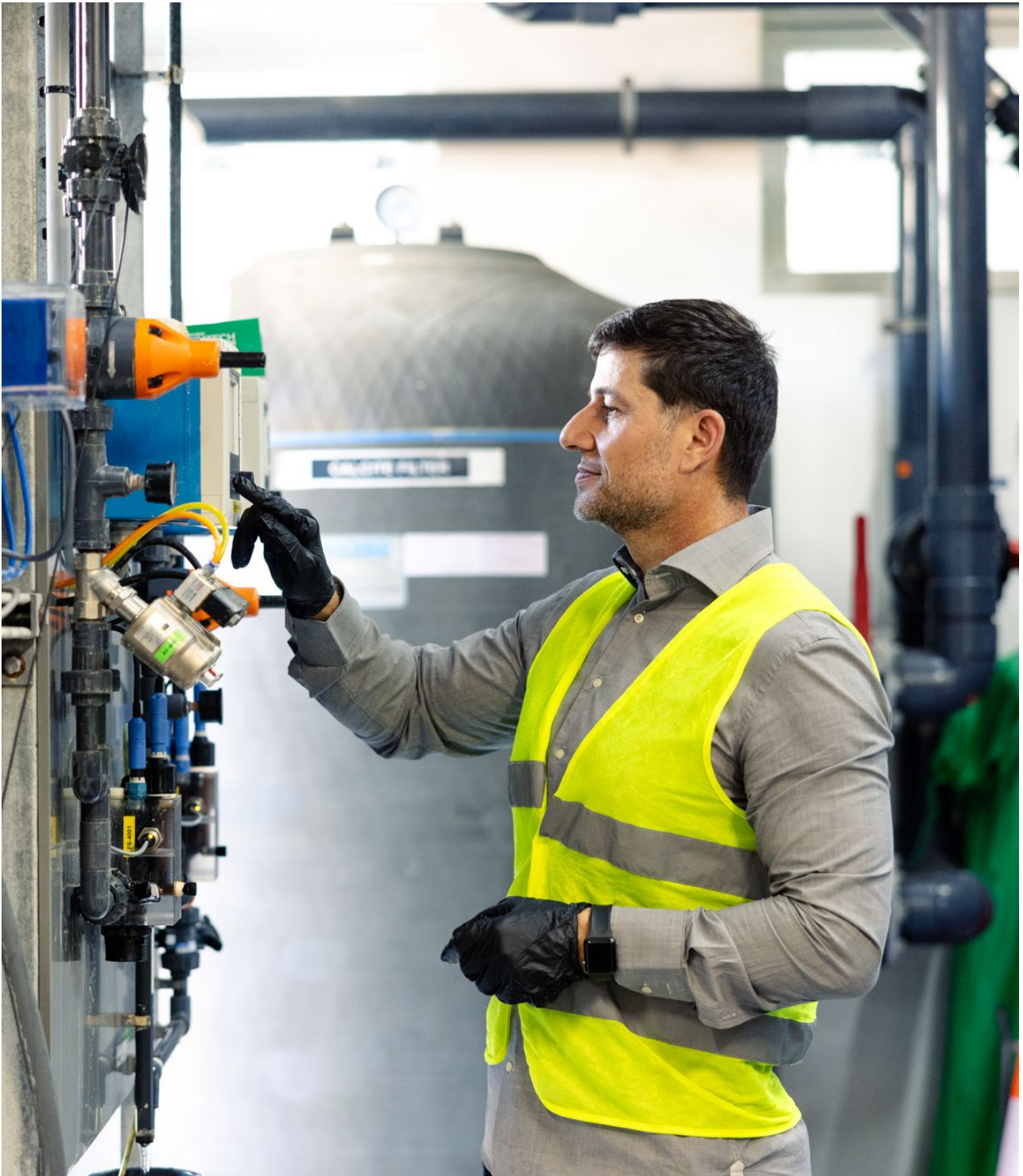
Image 4. Checking our water irrigation system. Chris Southwood/City of Sydney
